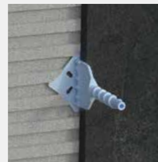
Linear leveler installation.
