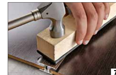
7) With the help of a wooden tapping block, apply pressure evenly over the whole length of the profile using a hammer. If tapping is done correctly, a "click" will be heard when the profile slots into place.
