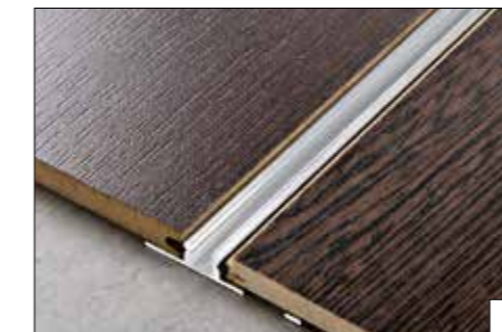
3) Lay the floor correctly leaving between 3 and 10 mm gap for the natural expansion of the wood.
