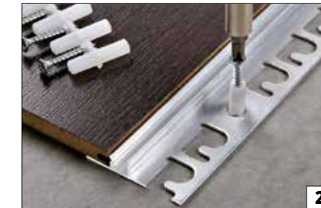
2) Fix and/or glue the base to the floor.
