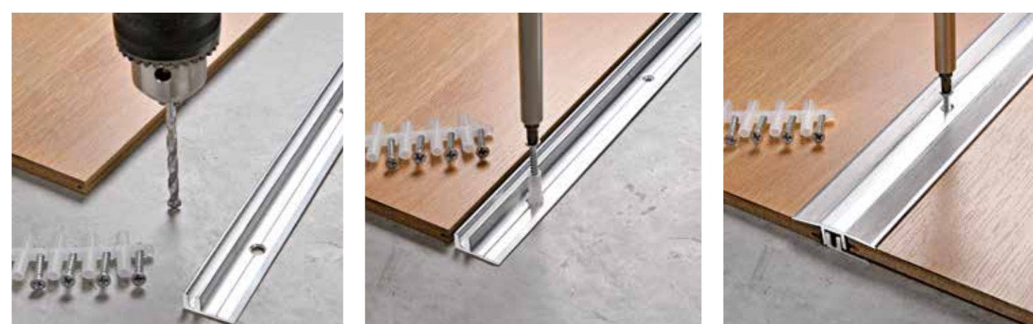
EXAMPLE OF LAYING
